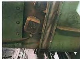
Combustion air pressure monitor
