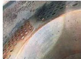
Reversing chamber - back end
