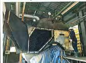
Front reversing chamber – Front door
