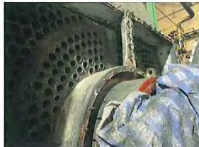
Combustion chamber / Rear access hole
