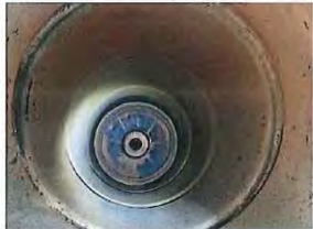
Reversing chamber - smoke tube 2 nd pass
