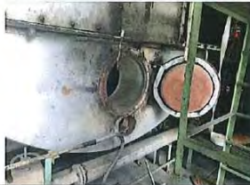
Reversing chamber - smoke tube 2 nd pass
