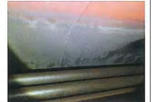
Reversing chamber - Flame tube / wet back
