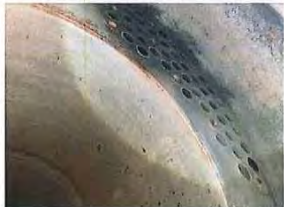
Rear door - smoke tube 3 rd pass
